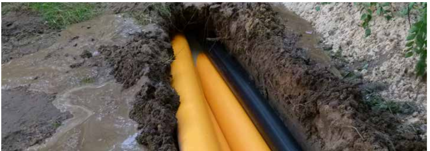
Gasleitung Coex d 160 mm, SDR 11 Gas pipe Coex d 160 mm, SDR 11
