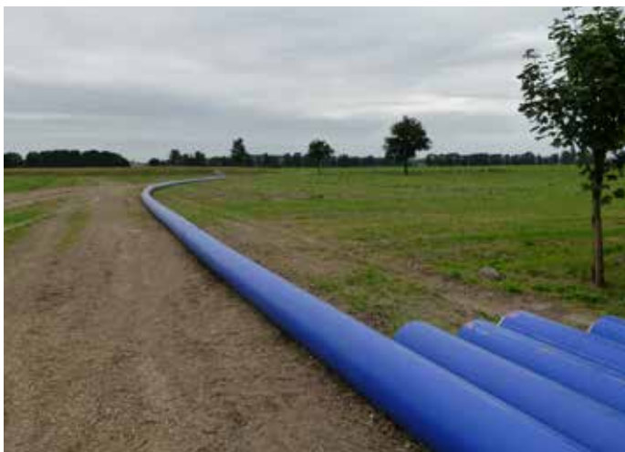
Trinkwasserleitung Coex d 450 mm SDR 17 Drinking water pipe Coex d 450 mm, SDR 17
